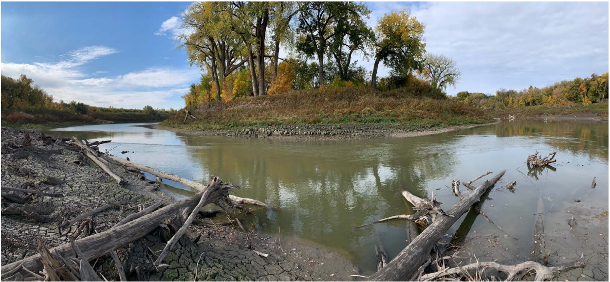
Figure 7. View across river showing fresh exposed and cracking sediments from material which was sent into and across the Red River from the slump
